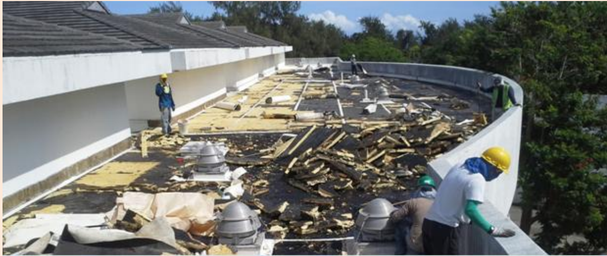
Roof Repairs Begin
